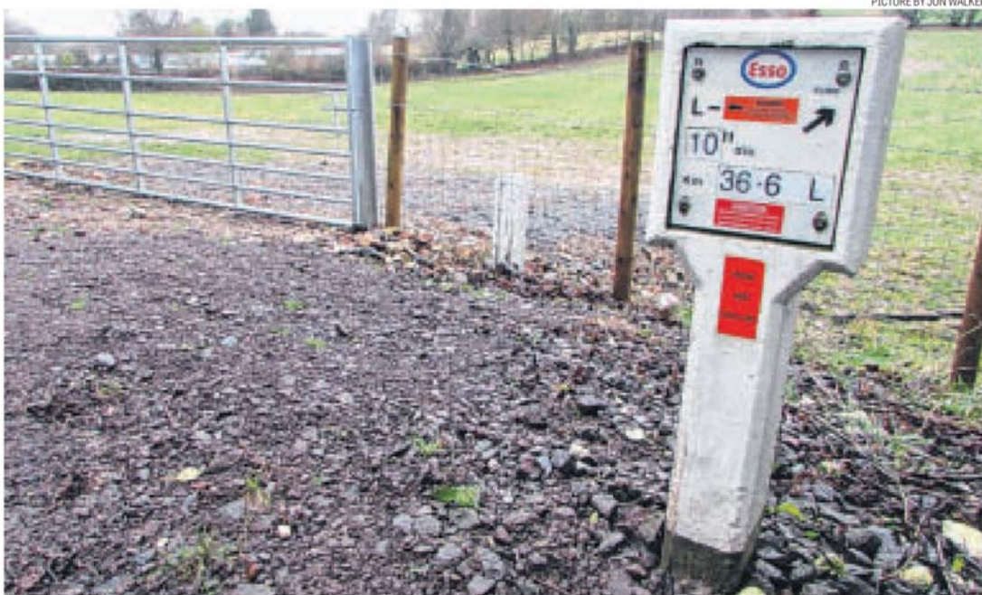
The new pipeline will run close to the route of the existing one – which is marked with sign posts like the one above where it passes through the Meon Valley.
